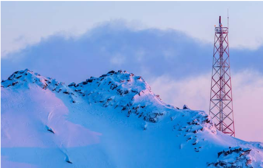
Telecommunication tower on the slope of a snowy mountain. Winter arctic landscape. View of the mountain top and the metal tower with antennas. Communication in the far north in the polar region.
