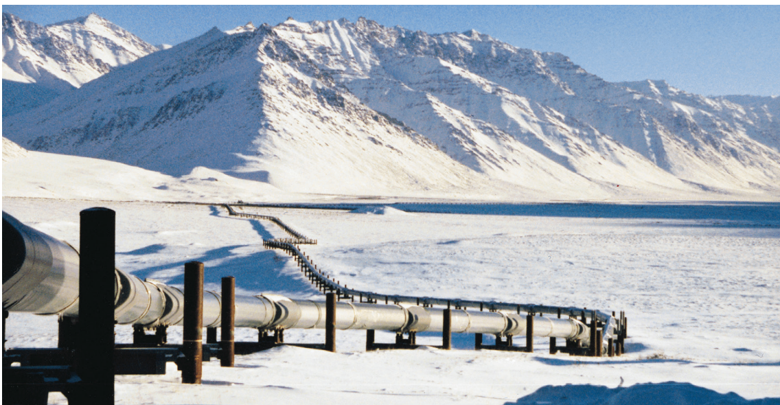
The Trans-Alaska Pipeline System (TAPS) moves oil from Prudhoe Bay to Valdez. With up to 1 billion bbls of potentially recoverable oil, more infrastructure will be necessary to unlock Arctic energy.
