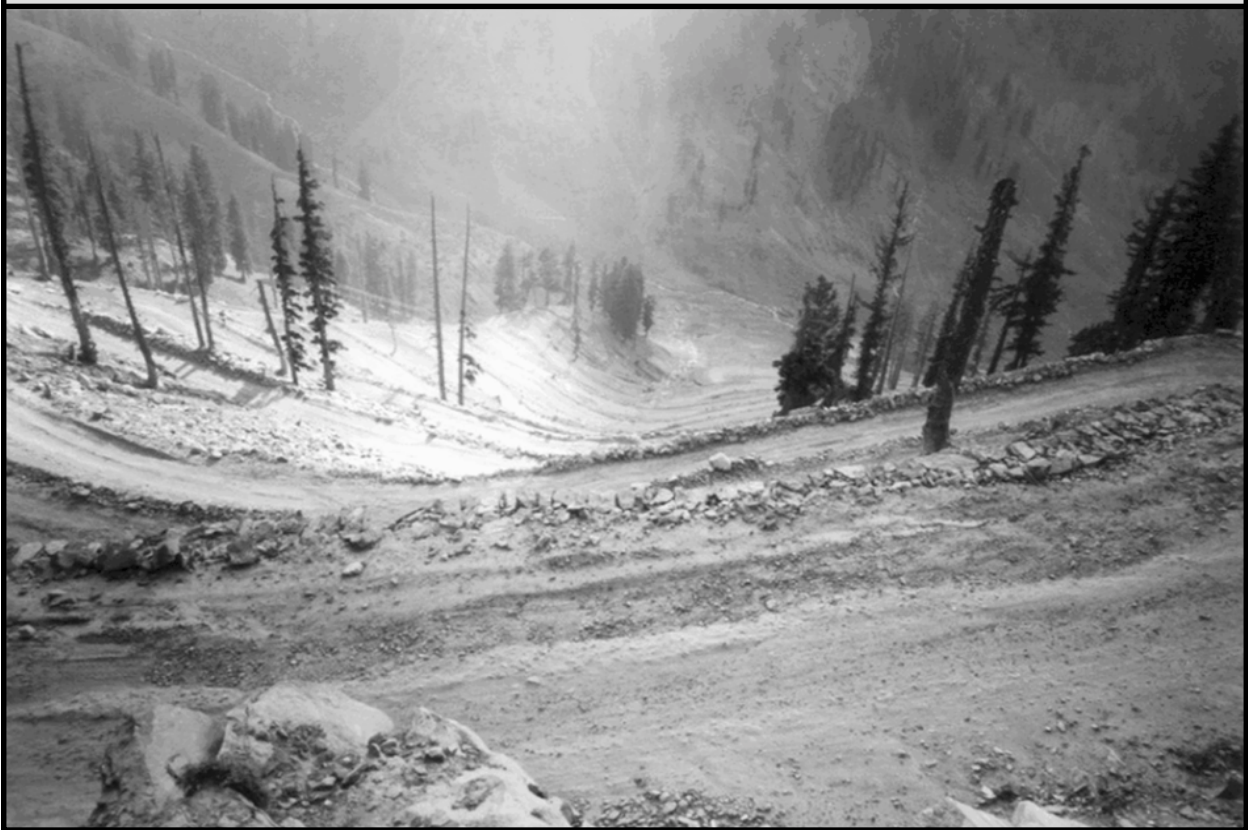
The road to the NWFP is highly vulnerable due to erosion and deforestation. (Photo by Richard Matthew).
