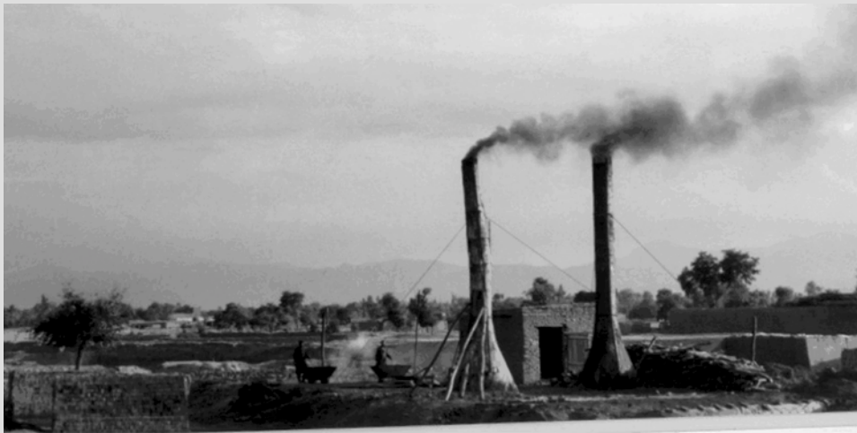
Brick kilns burning old car tires add to the high concentration of particulates in the air.
